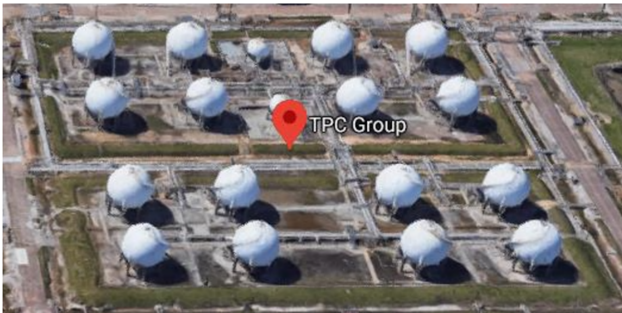
Figure 5: Aerial View of Select Storage Assets at PNO Terminal
