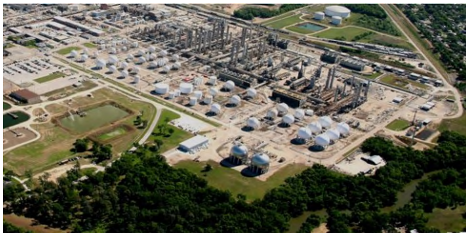
Figure 2: Aerial Photograph of HNO Facility
