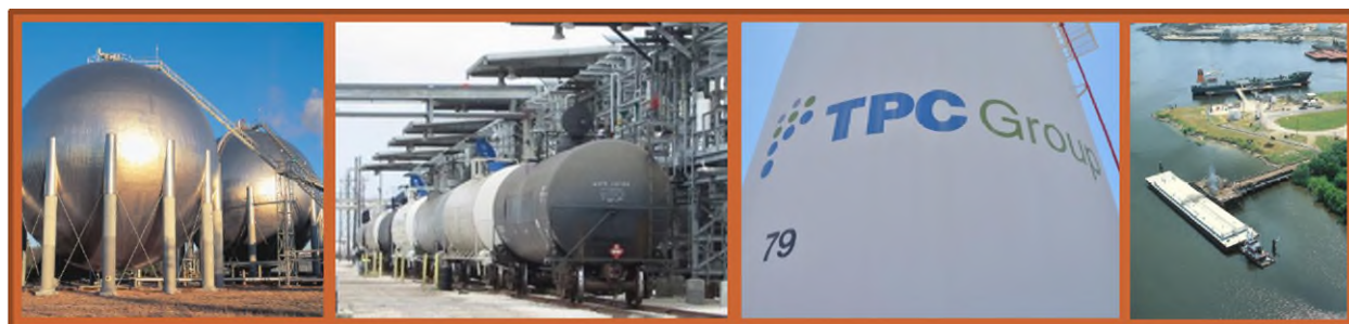
Figure 3: Terminal and Logistics Assets at HNO Facility
